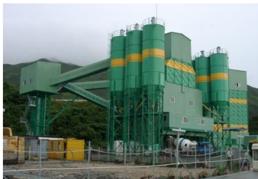
2个3立方米塔楼式搅拌楼 2X3 cubic meter Tower plant
